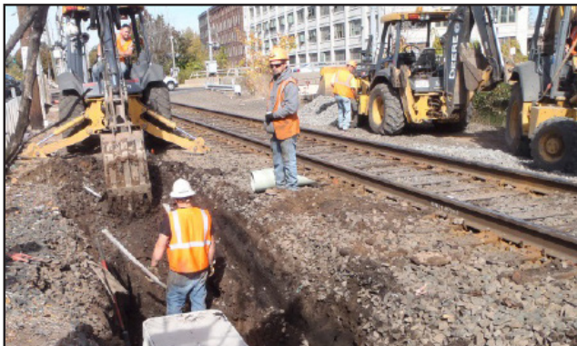
Installing innerducts and signal cable in Windsor Locks
